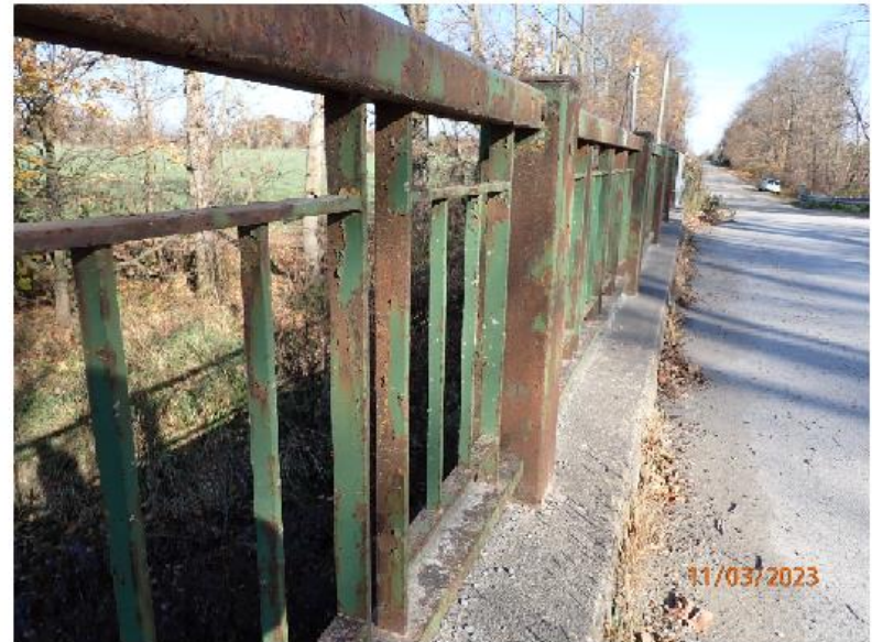
Photograph No. 4: 0418: Corrosion in railing (typ).
