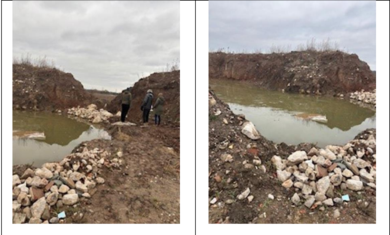
Berms located along the east side of the site and uncompleted stormwater works.
