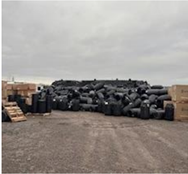
Looking south into the site with new delivery of rain barrels/composters to be assembled with the lids and stored.
