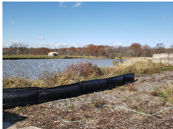
Figure 4 - Silt Fence Protection Along Pond
