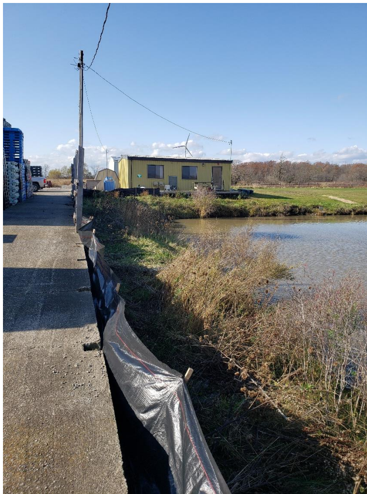
Figure 5 - Silt Fence Installed at the Request of NPCA and Niagara Region
