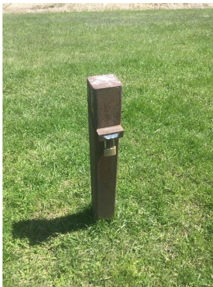
Figure 1 - Example of a stick-up protective casing for a monitoring well
